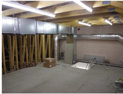
Loft storage space
