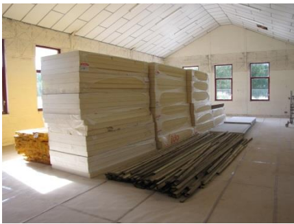
Insulation waiting to go up
