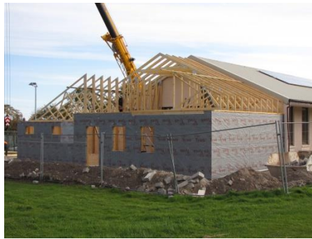
Building the extension
