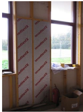
Lining the walls
