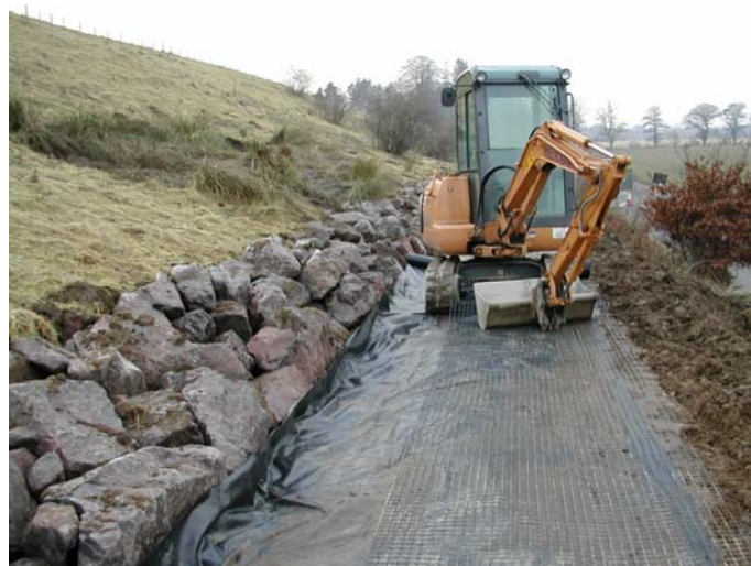
Construction of the new path
